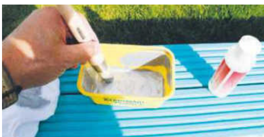
A sparse amount is needed; a small squirt of Extender allows for a longer working time
